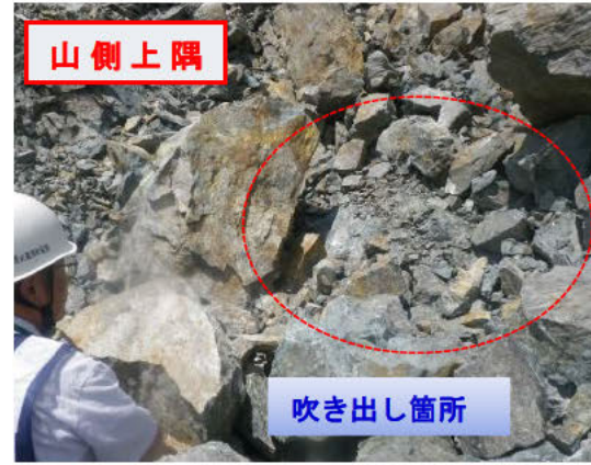
切羽 (山側状況)
